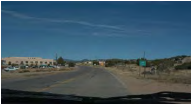
Looking north along NM 4 at the entrance to the Pueblo of Jemez. NM 4 is predominantly a two-lane rural road with wide shoulders, with a speed limit of 30 mph along this segment.
